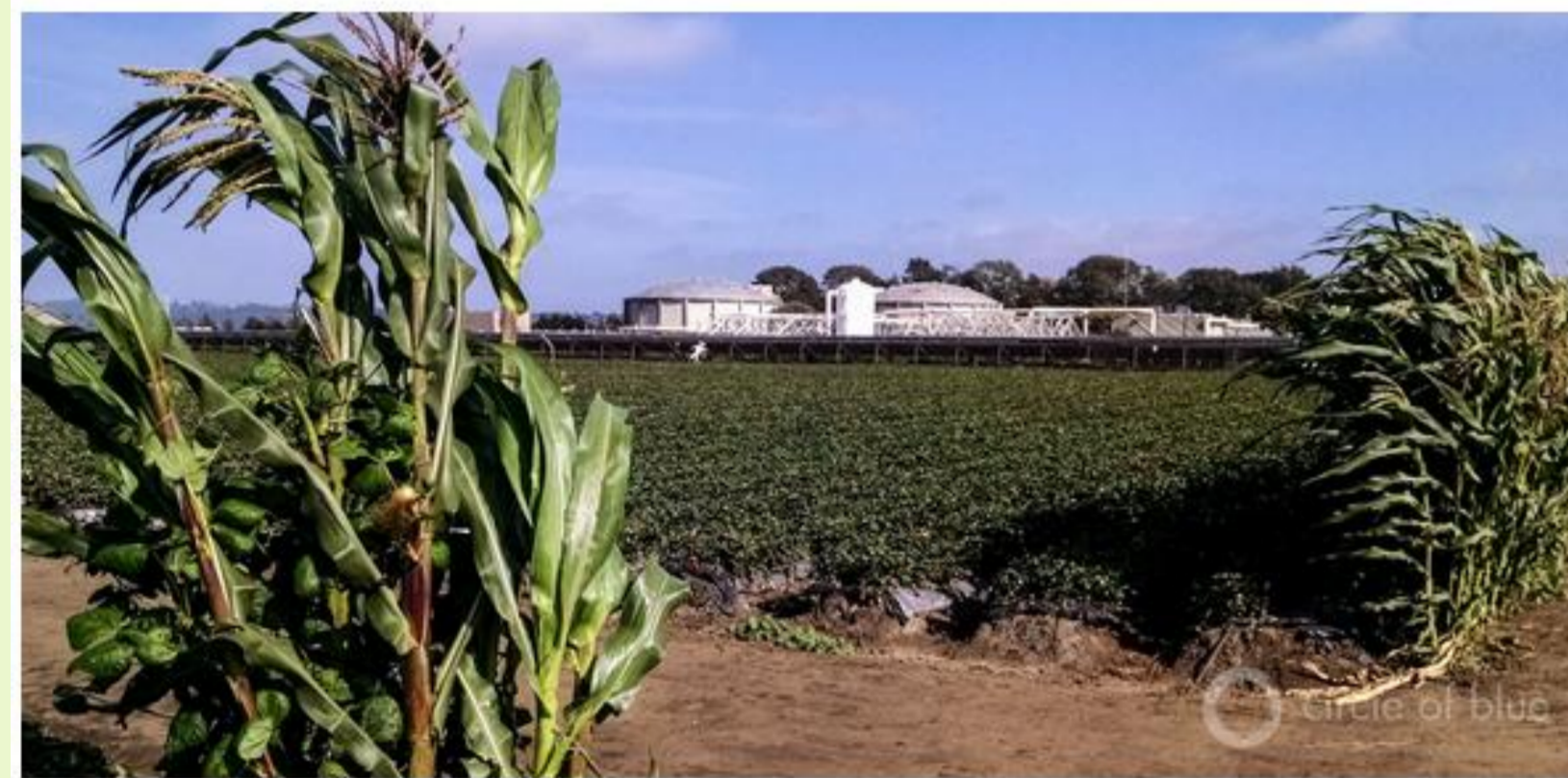
The Watsonville, California, recycled water facility, completed in 2009, purifies wastewater from the city of Watsonville for use by farmers in the Pajaro Valley. Using recycled water instead of groundwater prevents the Pacific Ocean from spoiling coastal aquifers with salt. Click image to enlarge.
