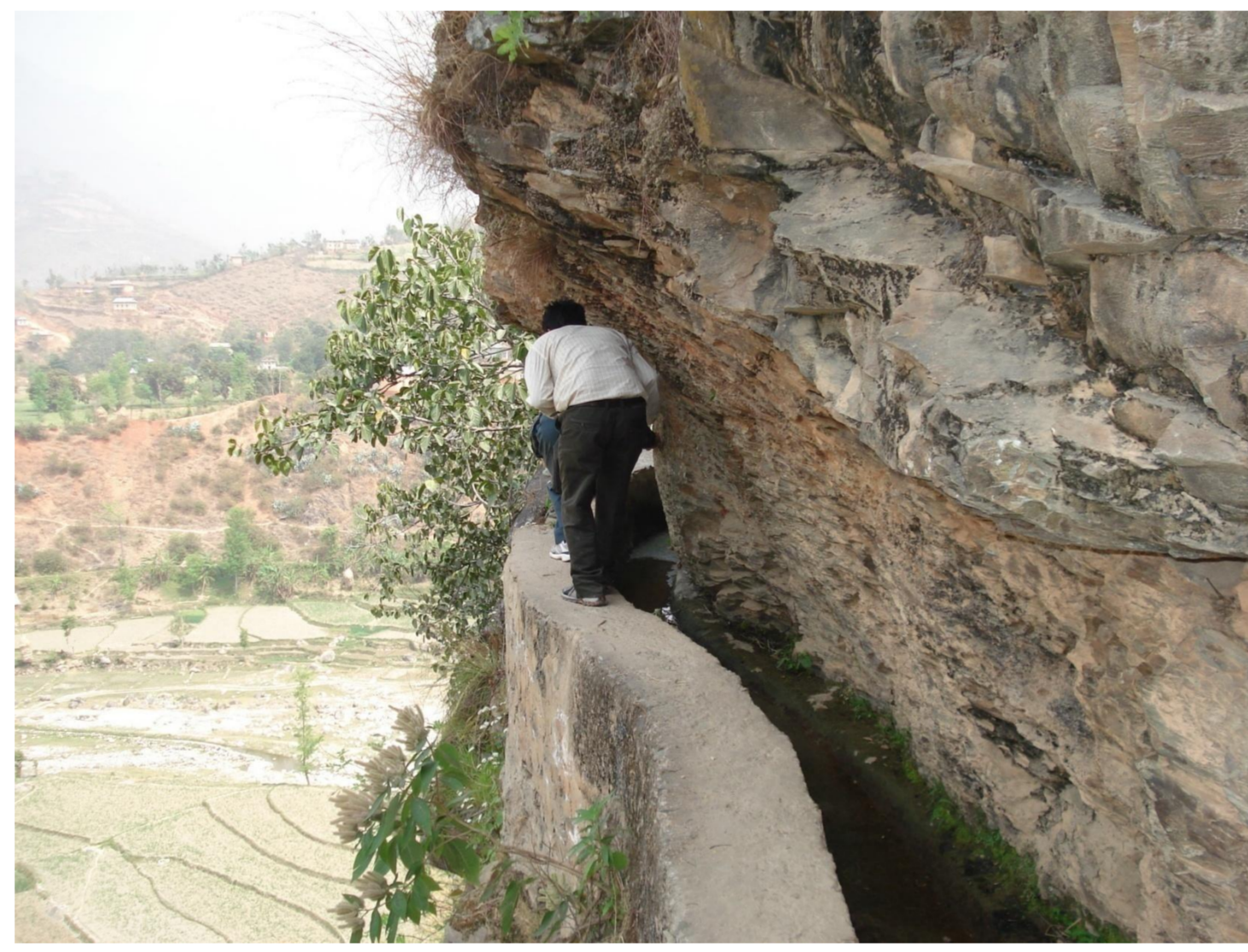
Semi tunnel section with stone masonry lining
