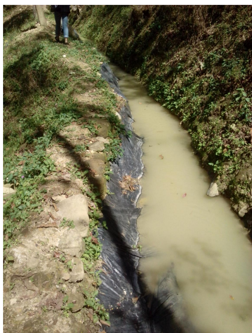
Polythene sheet laid to check seepage loss
