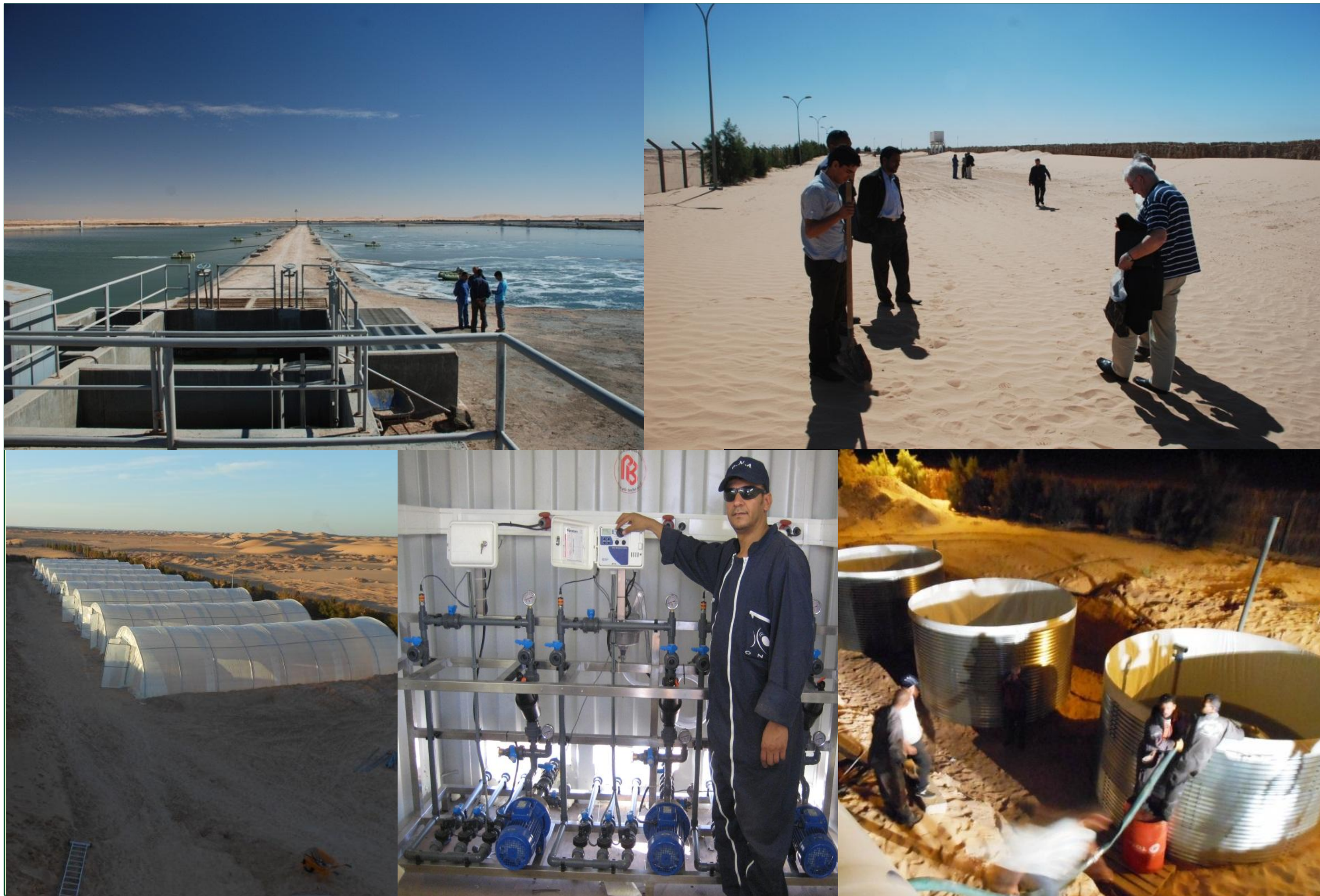
Existing Waste water treatment work (aerated lagunes), agro-site (before), greenhouses (after), Irrigation system, water tank for 3 water quality
