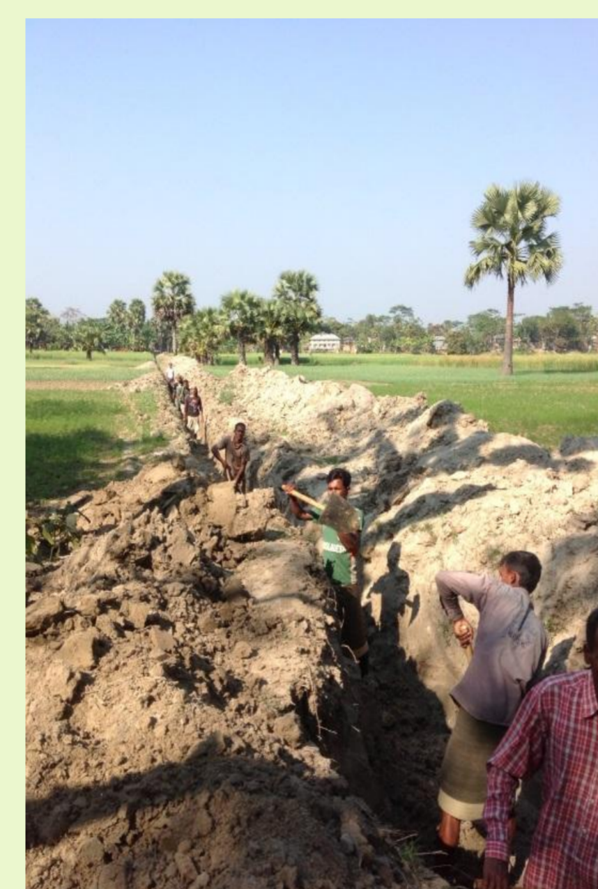
Excavation of trench for buried pipeline
