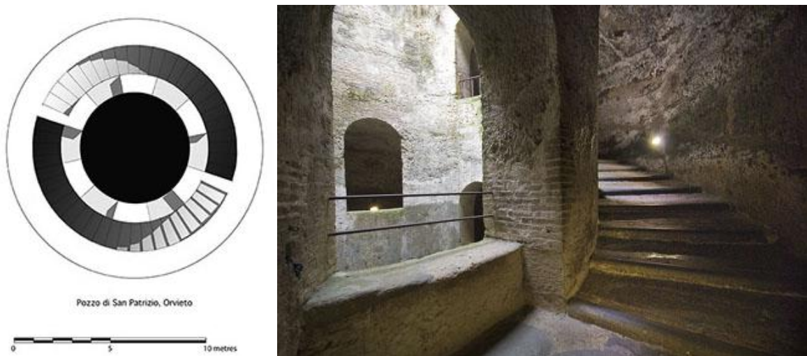
Figure 1 Spiral staircase in S. Patrick well, Orvieto, Italy
