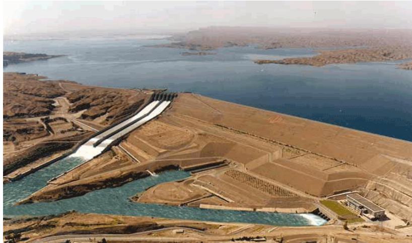
Figure 1. A general View of Karkheh dam
