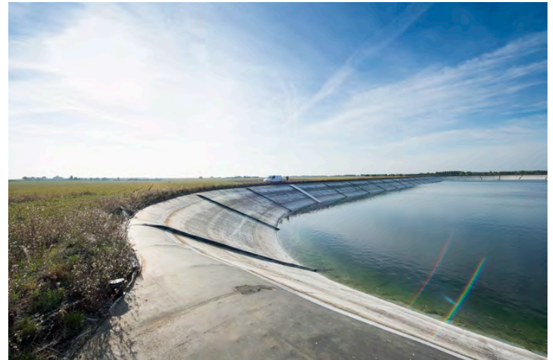
Infrastructure development in 2010
